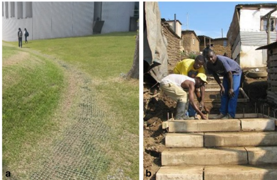
Fig. 6 Trail surface reinforcement and upgrading: a Keio University, Fujisawa, Japan; b Redcliffe informal settlement, eThekweni, South Africa (source: [80])
